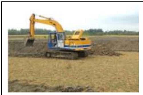
Use of Excavator in Sorjon Plot
