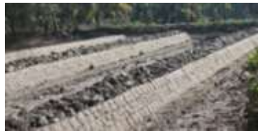
Manual Excavation in Sorjon at CN
