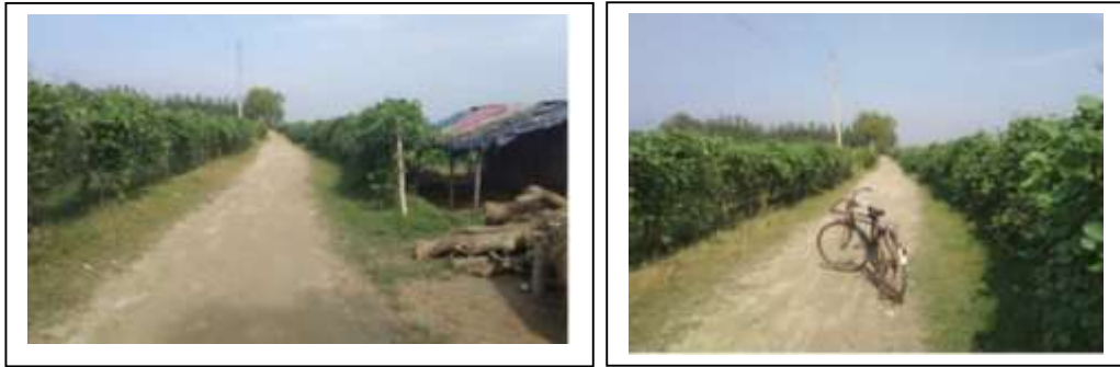
Earthen road from Montaz Khali to Ziller khal river bank
