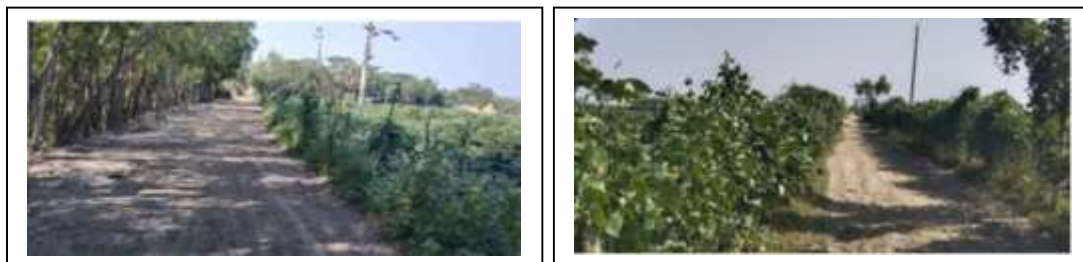
Golapi market Embankment to Eusuf Prof. project Meghna River bank
